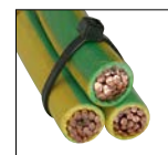
Nylon cable tie tensioned and cut i.e. no sharp edges
